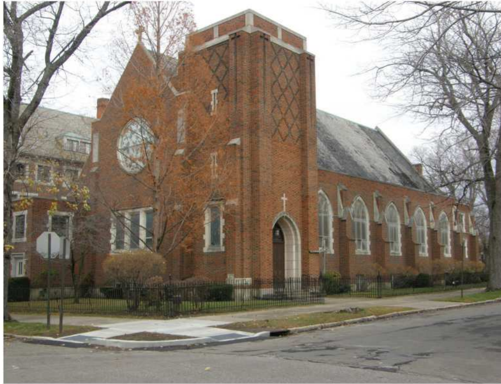
Plum Street and West 9 th Street - Southwest Elevation
