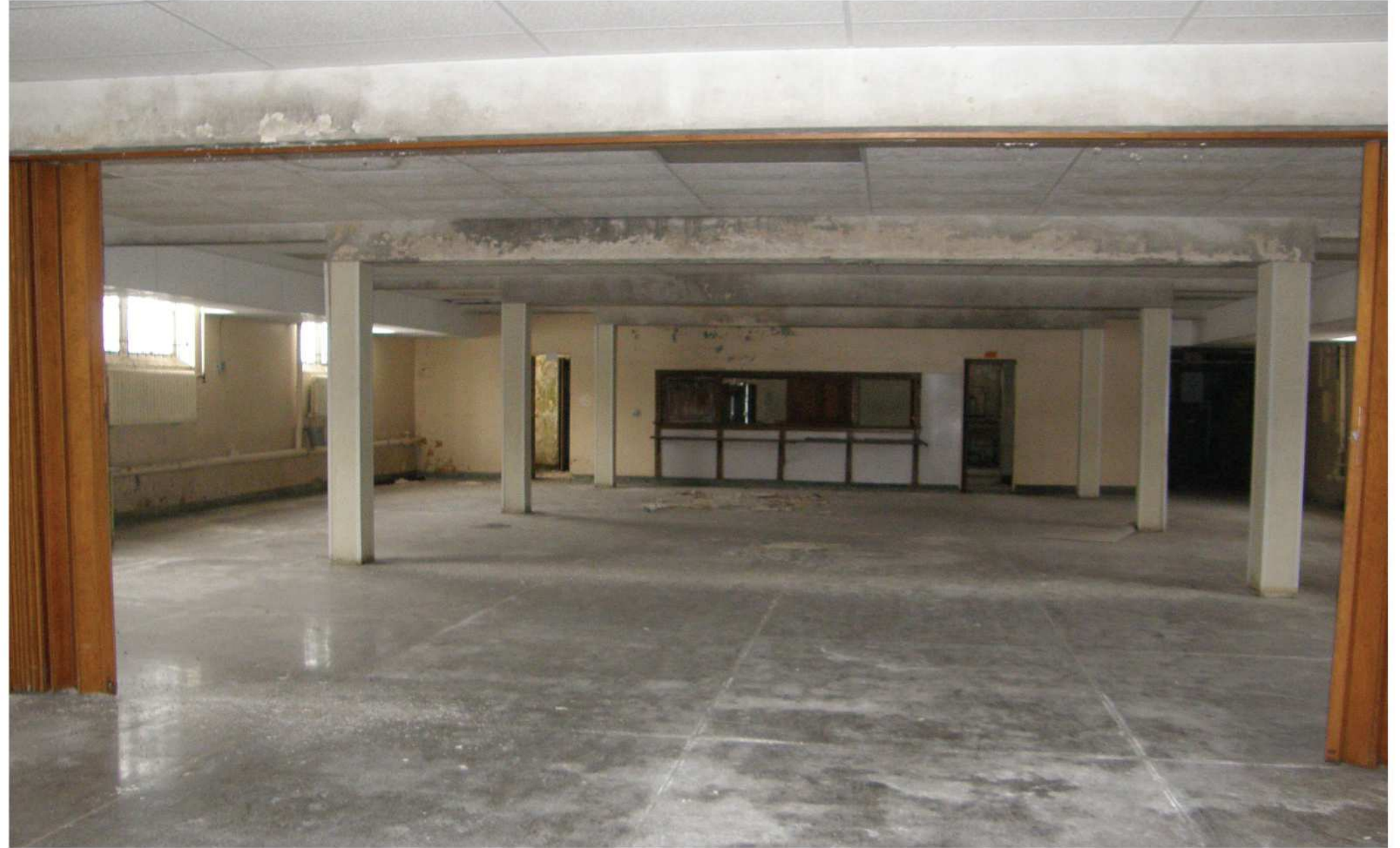
View of Basement Dining Room Looking West
