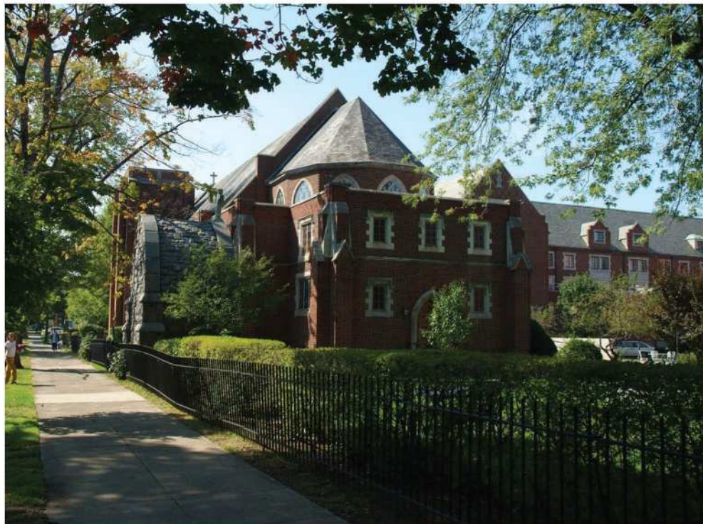
West 9 th Street - Southeast Elevation
