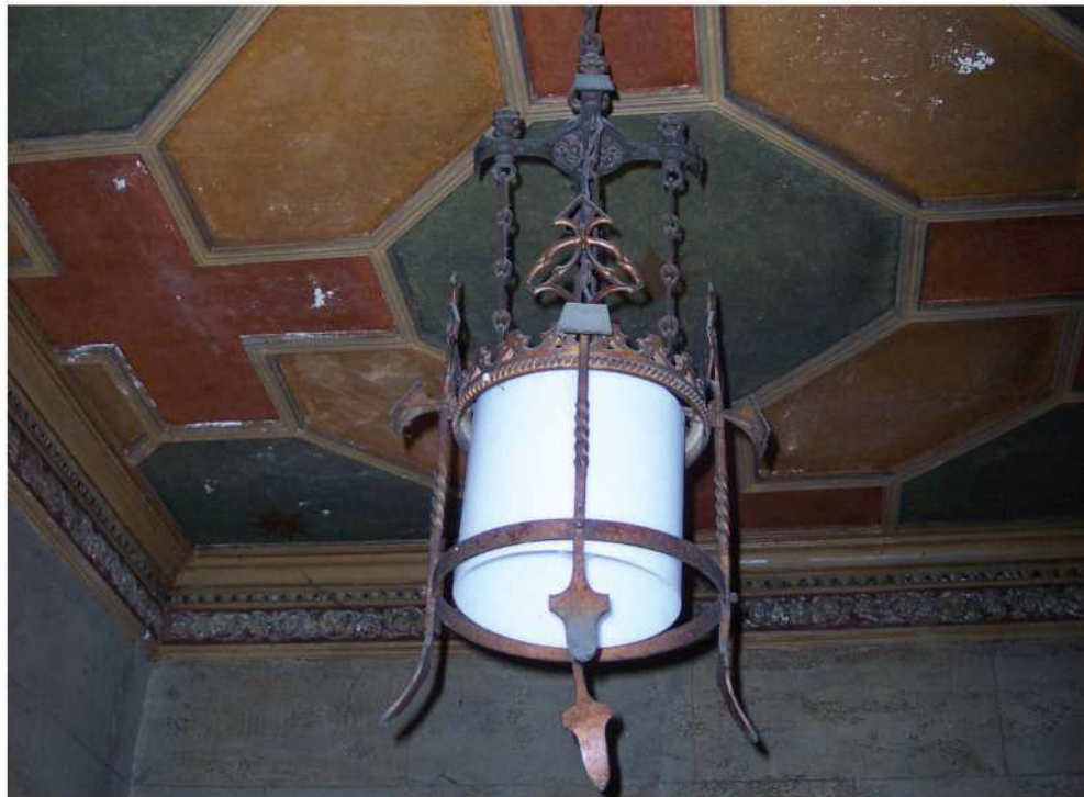
View of Ceiling Detail and Light Fixture
