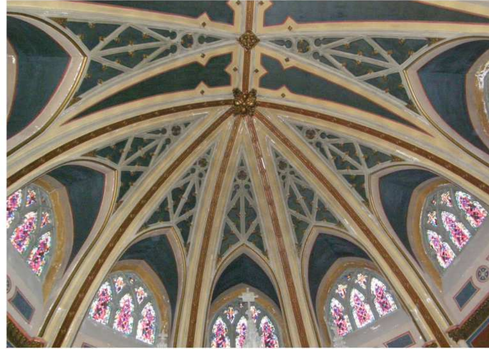
View of Sanctuary Ceiling
